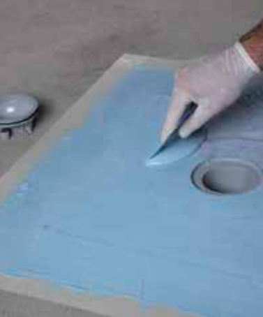
Impregnating Drain Vertical fabric with Mapelastick AquaDefense
