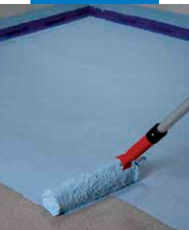
Application of the first coat of Mapelastick AquaDefense on a screed
