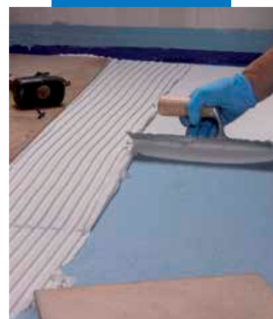
Bonding tiles on Mapelastac AquaDefense
