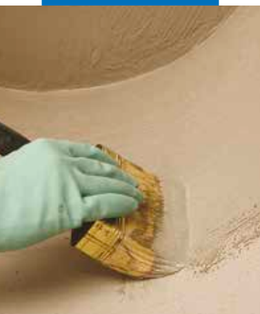
Waterproofing of details by brush
