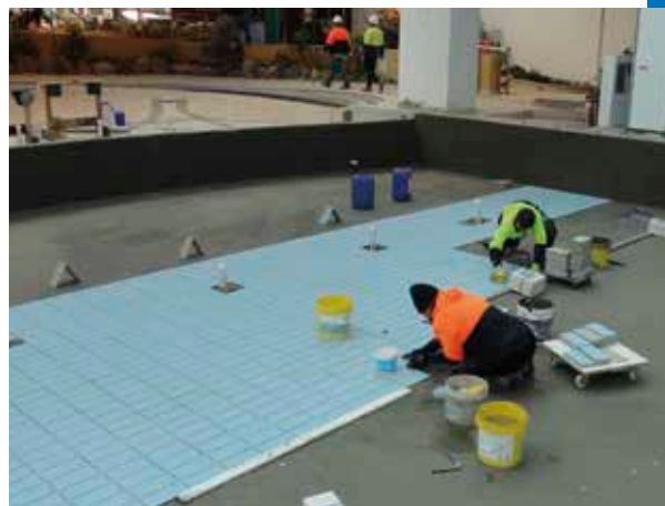
Installing pool tiles over Mapelastic Smart waterproofing membrane
