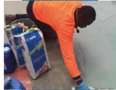
Installing Mapelastic Smart in the 50 metre pool at the Adelaide Aquatic Centre
