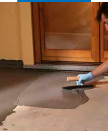
Waterproofing of terraces by trowel
