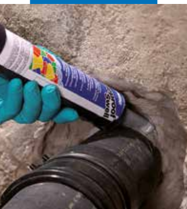
Applying Mapeproof Swell around a pipe
