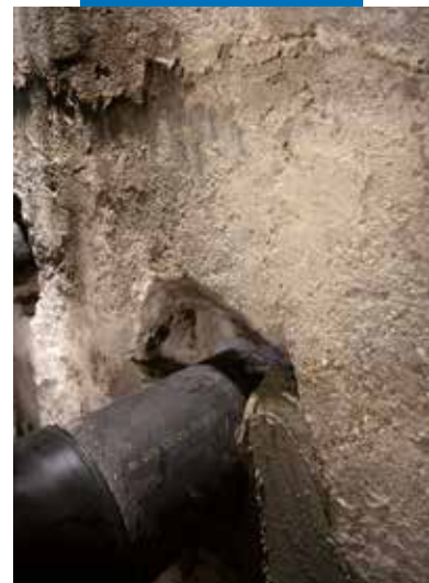
Confining Mapeproof Swell with a product of the Mapegrout line
