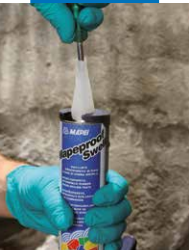
Piercing the protective membrane on the Mapeproof Swell tube
