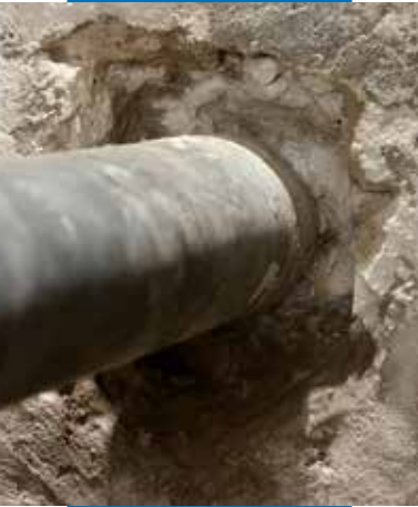
Breaking out structure around a pipe
