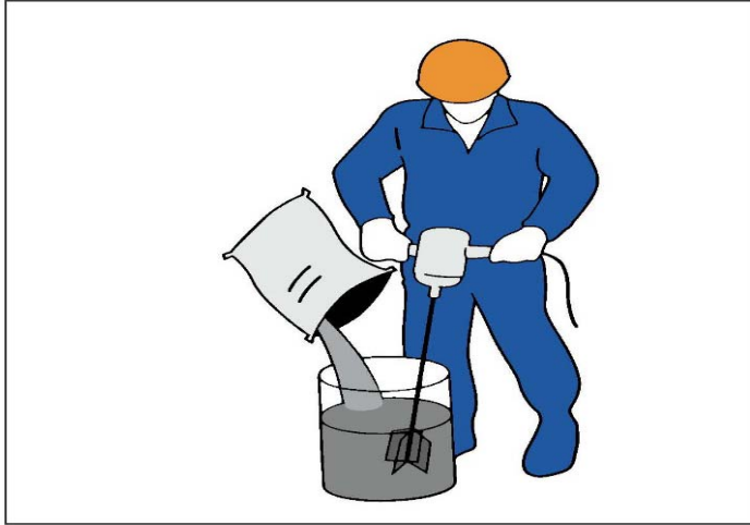
Figure 1: Mixing the grout with a birdcage paddle on the mixer
