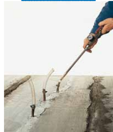
Restoring horizontal structure by injection with Epojet
