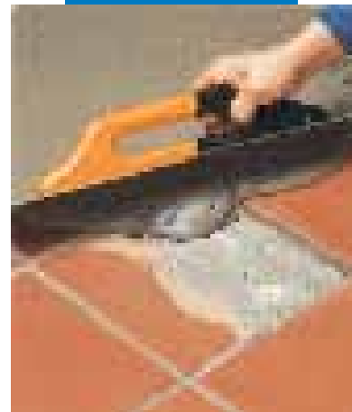
Filling holes with Nivorapid
