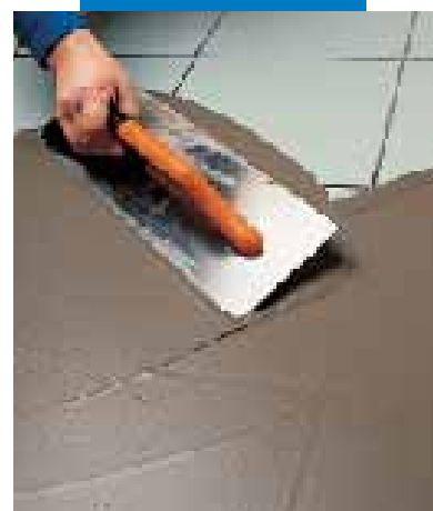
Levelling of existing floor with Nivorapid
