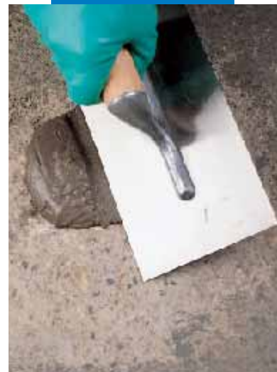
Repairing horizontal joints with Nivorapid
