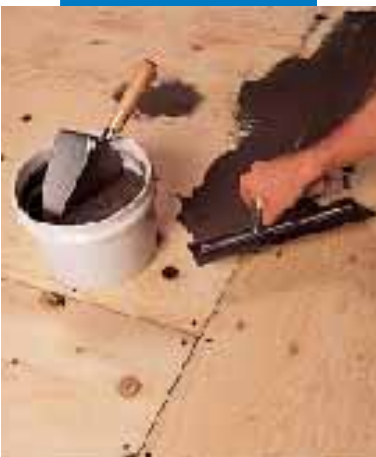
Grouting a plywood substrate with Nivorapid + Latex Plus
