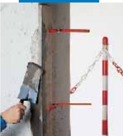
Repairing vertical arrise with Nivorapid
