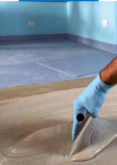
Applying Ultrabond Eco 380
