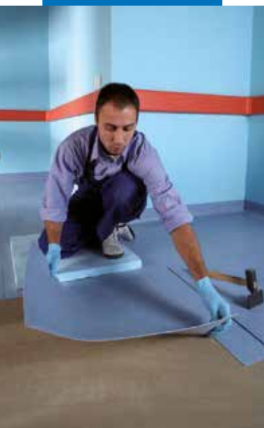
Installing PVC floor tiles
