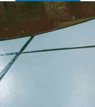
Application of Ultraplan with a metal trowel on an existing ceramic tile floor after the application of Eco Prim T Plus
