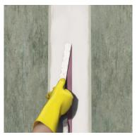
Apply the Combiflex SG tape within the open time of the adhesive. Press the tape firmly, without trapping air, into the adhesive using a suitable roller. The adhesive should be squeezed out on both sides of the tape by ~5 mm.
