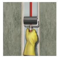
Let the first layer of the Sikadur<sup>®</sup>-31 begin to harden before the top layer is applied. Apply the top layer of adhesive at a thickness of  $\sim$  1 mm on both sides of the joint / crack, producing a fully covering layer which tapers outwards to almost zero.
