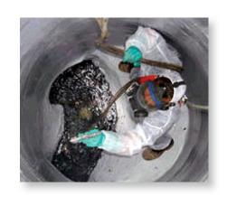
sulphuric acid as a waste product which then attacks the substrate. This sulphuric acid will quickly destroy ordinary concrete-based materials in a municipal sewer system.
