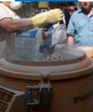
Preparation of Ultratop in a mixer
