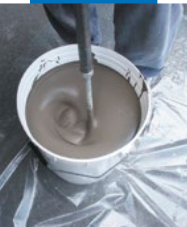
Preparation of the product with a drill
