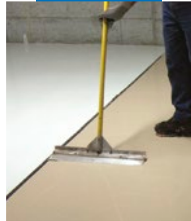
Smoothing Ultratop immediately after spreading
