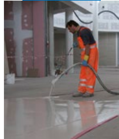
Mechanical application of Ultratop
