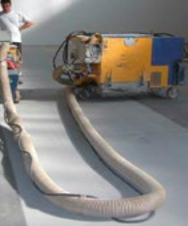
Preparation of the substrate by shot-blasting
